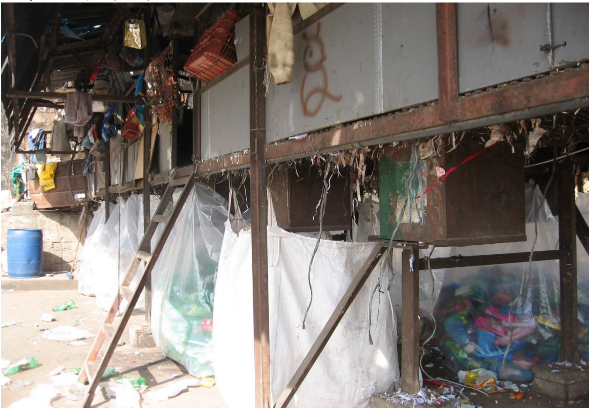
Figure 11. COOPERT: underneath the structure of the conveyor belt. Bags positioned to receive sorted items. Source: R. Perrupato-Stahl, C. (2014)
