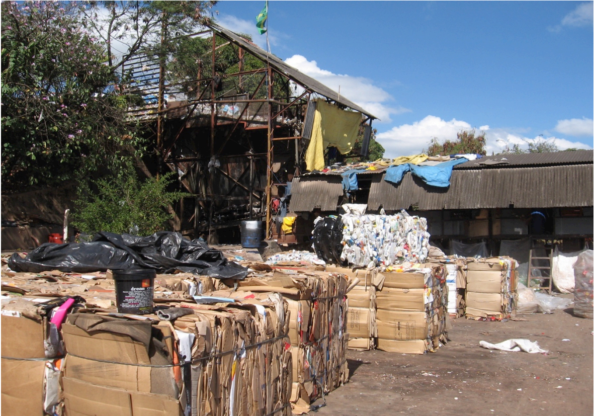
Figure 10. Outside view of COOPERT's sorting facility. Conveyor belt beneath the roof. Source: R. Perrupato-Stahl, C. (2014)
